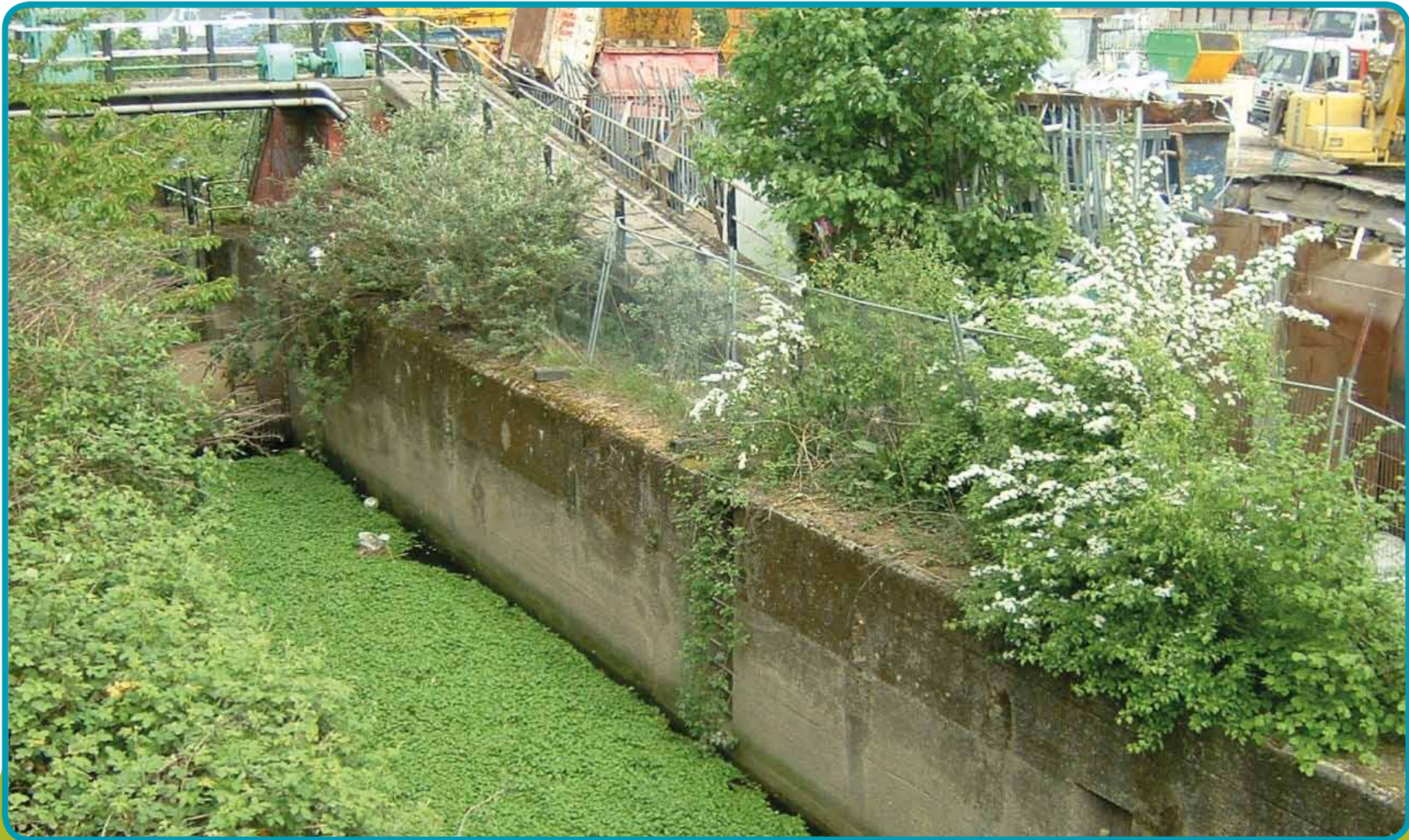
Carpenters Road Lock in 2008.
