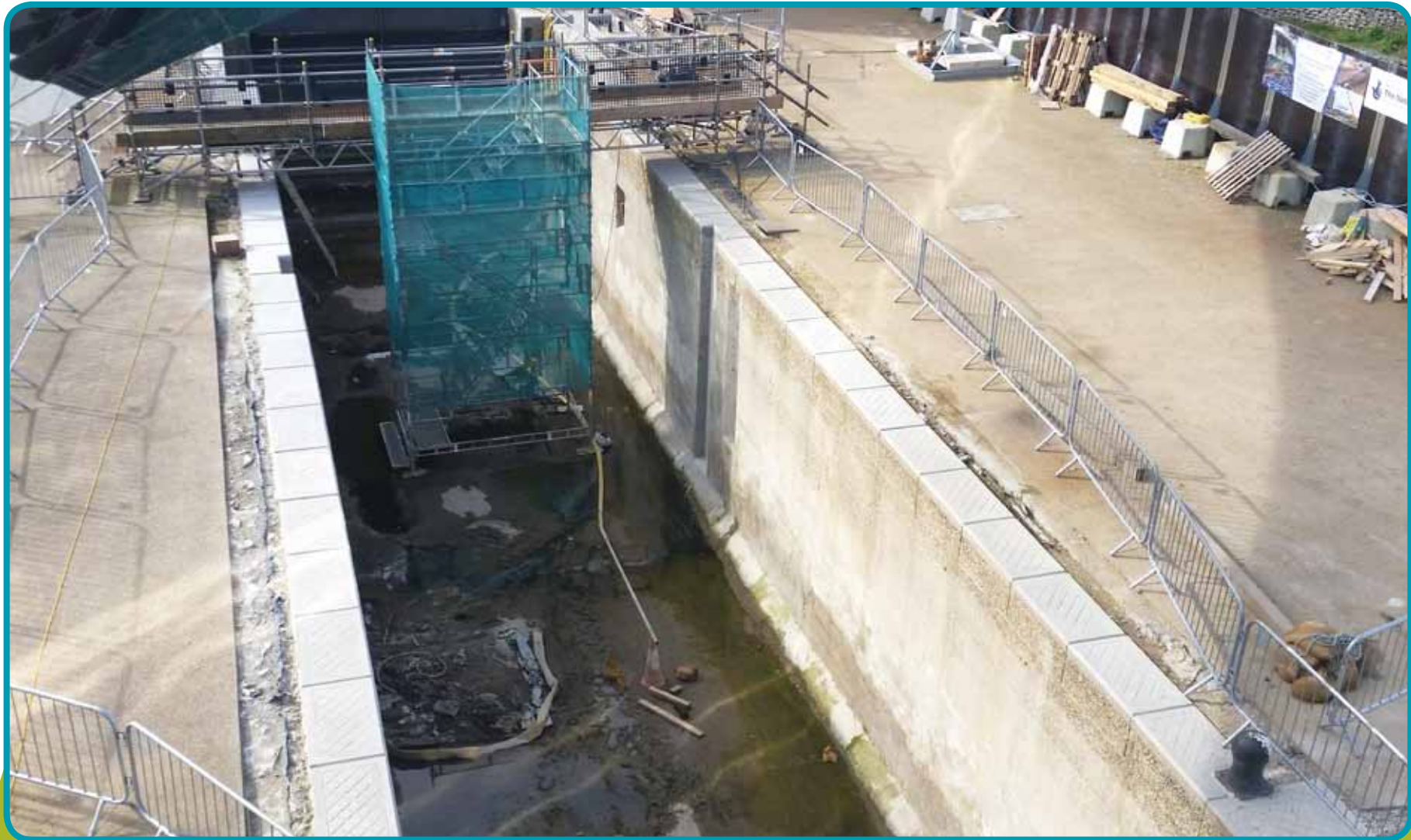
Draining the lock, 2017.
