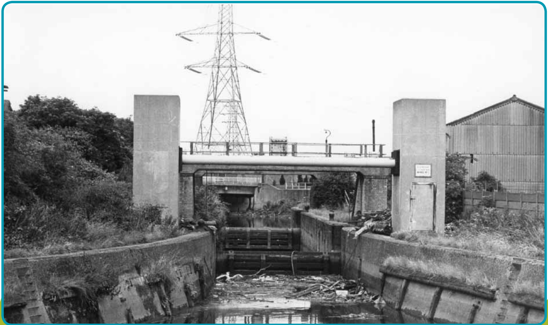
Carpenters Road Lock in the 1970s.
