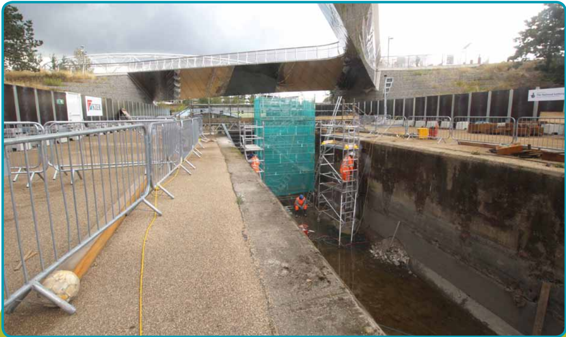
Repairing the lock walls, 2017.
