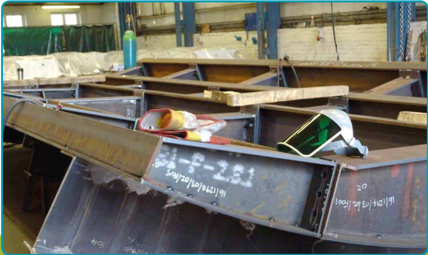
Building the new radial gates in Sheffield, 2017.
