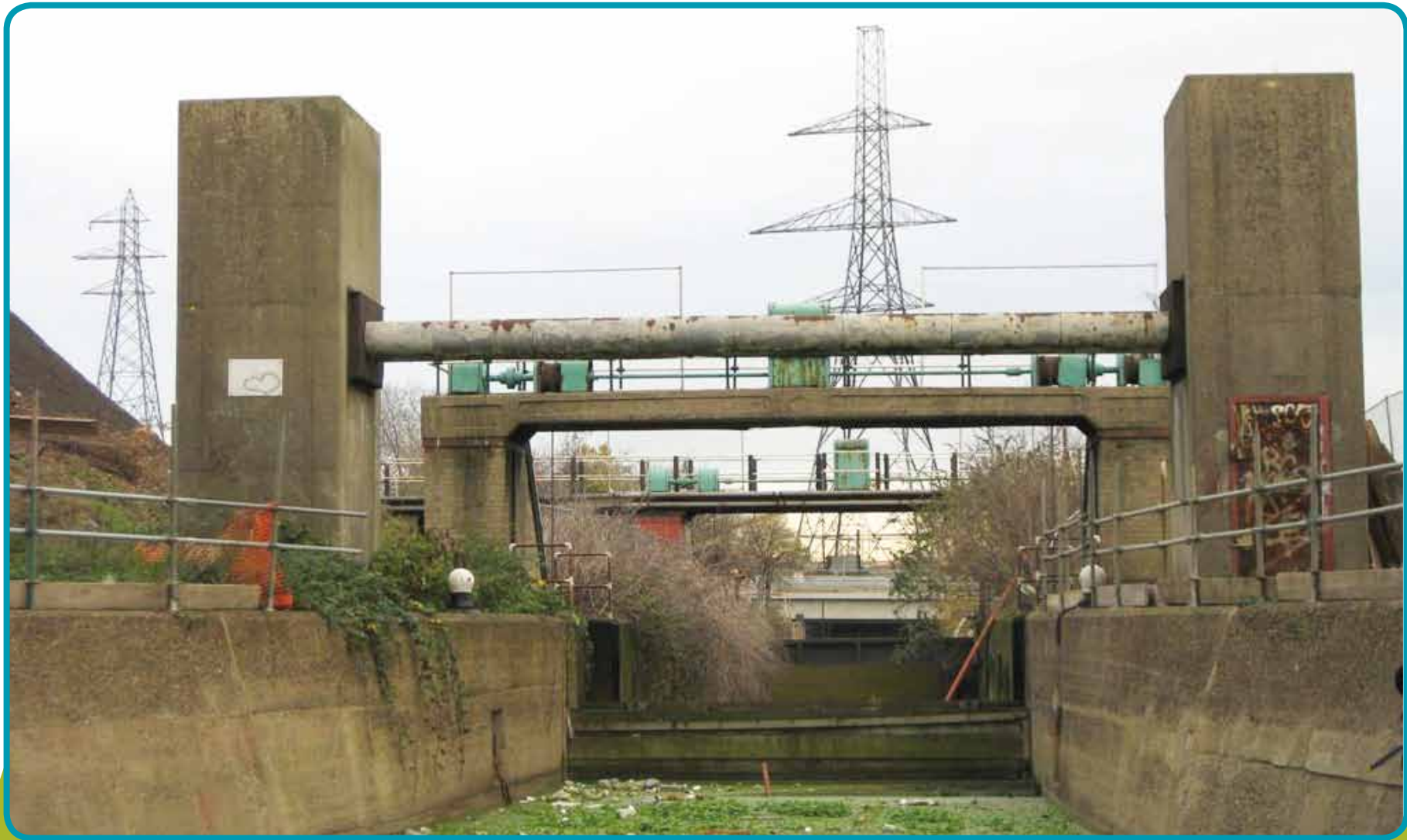
Carpenters Road Lock in 2008.
