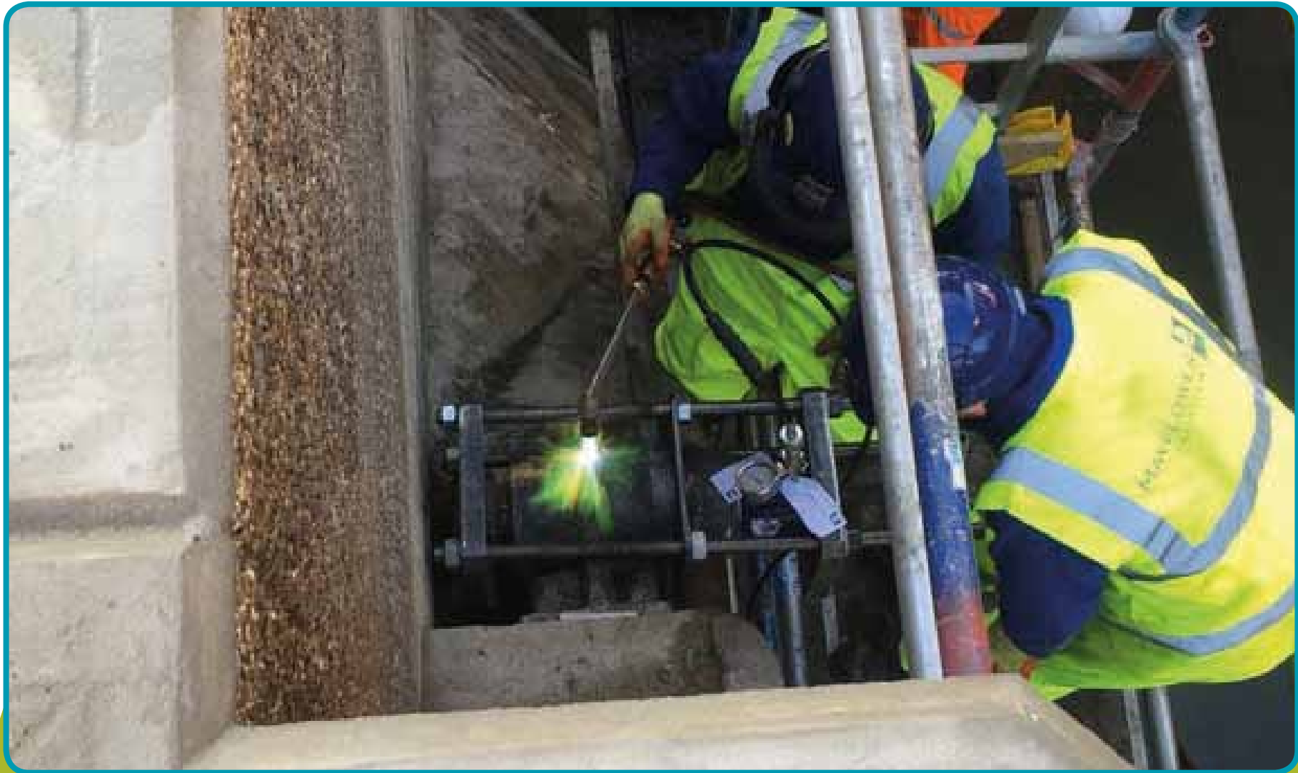
Replacing the radial gate pivot points, 2017.
