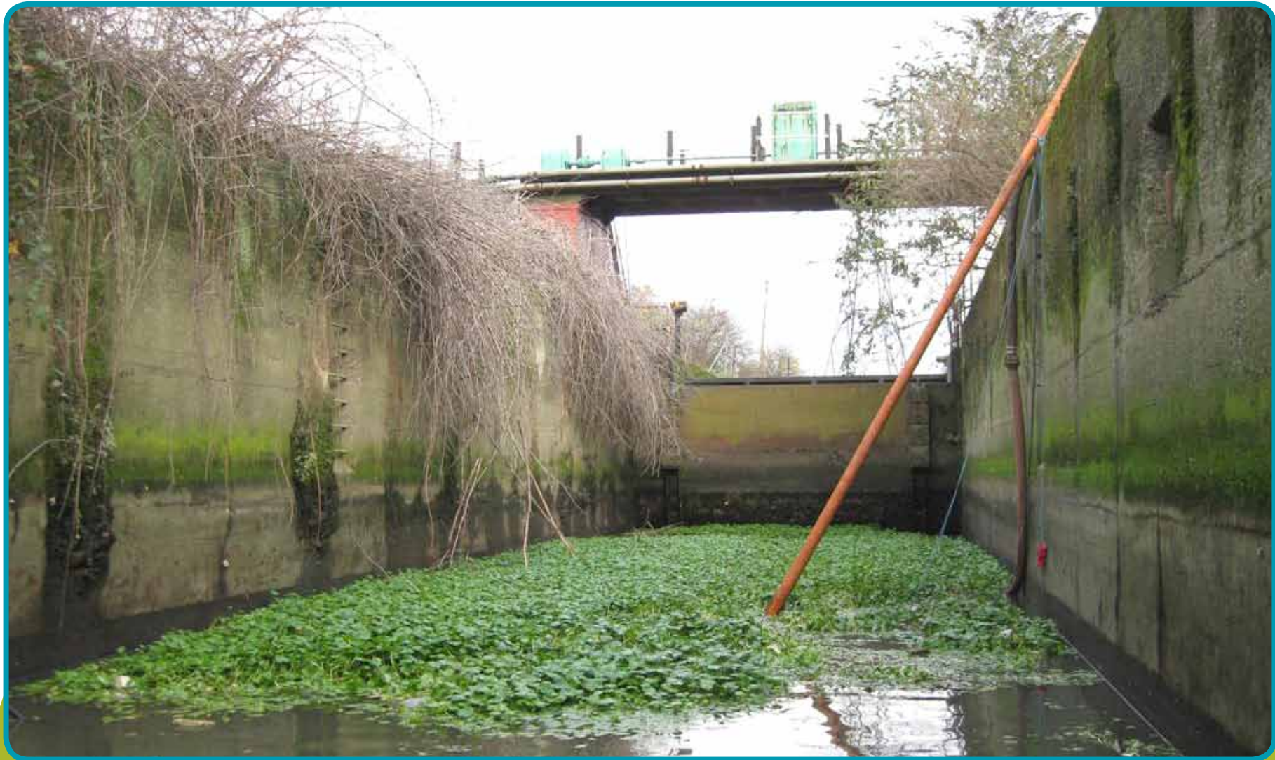
Inside Carpenters Road Lock in 2008.
